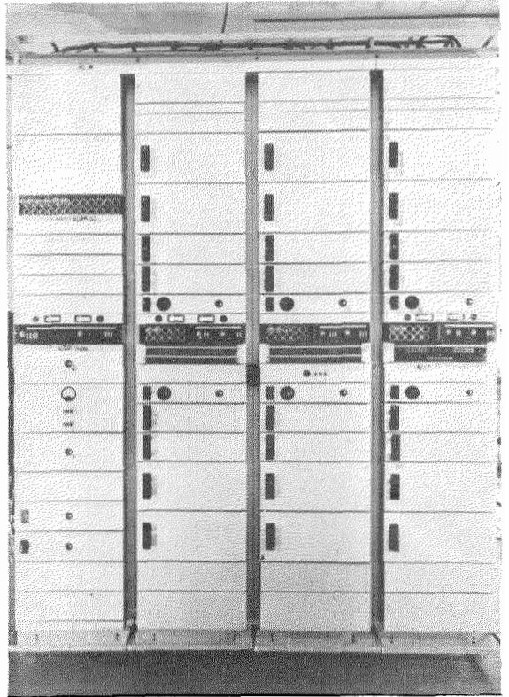
Fig. 13—Bay Containing Equipment for Six Carrier Channels.
