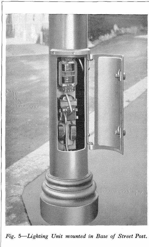
Fig. 5—Lighting Unit mounted in Base of Street Post.
